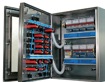
Zone 2 field station with front components and protective screen
