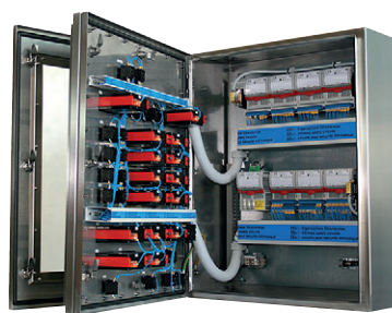
Zone 2 field station with front components and protective screen
